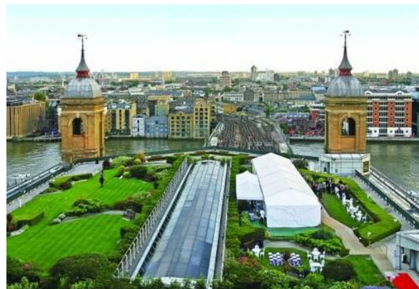
Slika 80: Cannon Bridge roof garden; London
