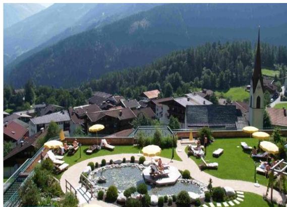
Slika 76: Zelena streha hotela na Tirolskem Vir: http://www.fbb.de/en/green-roof/fbb-green-roof-of-the-year/ , 15.11.2012
