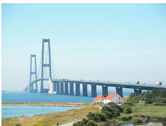
Slika 24: Most The Great Belt Bridge
