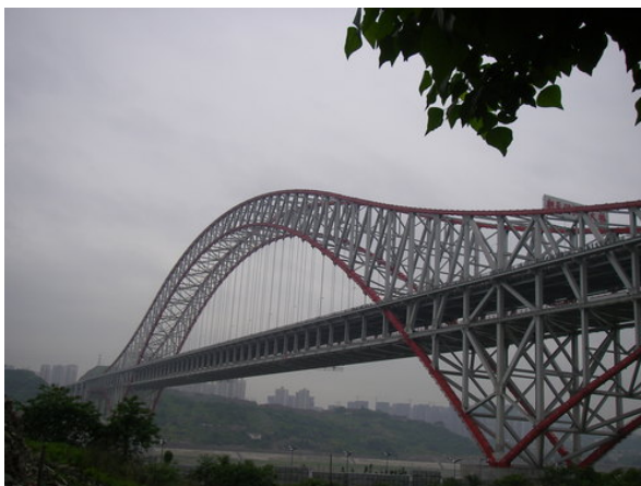
Slika 28: Most Chaotianmen Bridge
