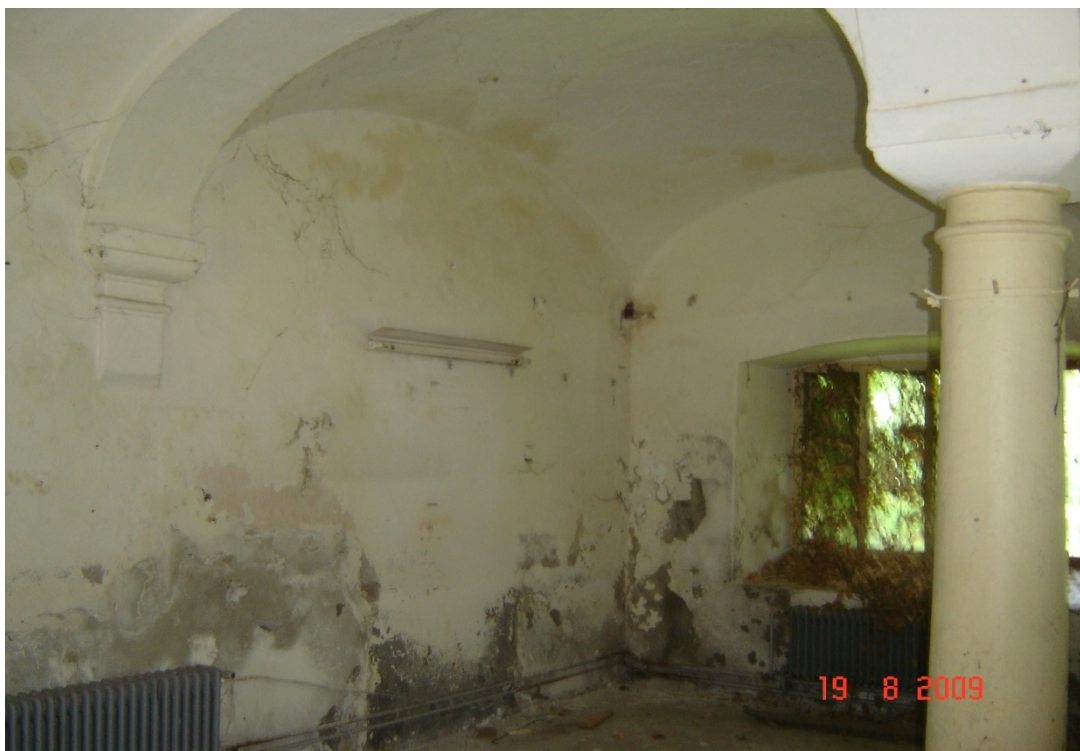
Slika 13: Vlaga v stenah in obokih
