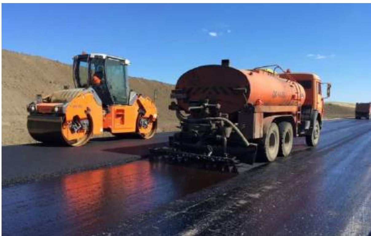
Slika 16: pobrizg z bitumensko emulzijo Vir: https://ibuilders-sl.techinfus.com/bitum/emulsiya/
